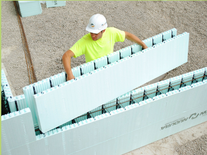
With R-values as high as R-48, Nudura Plus+ Forms can be assembled quickly and easily onsite, for optimal energy performance.
